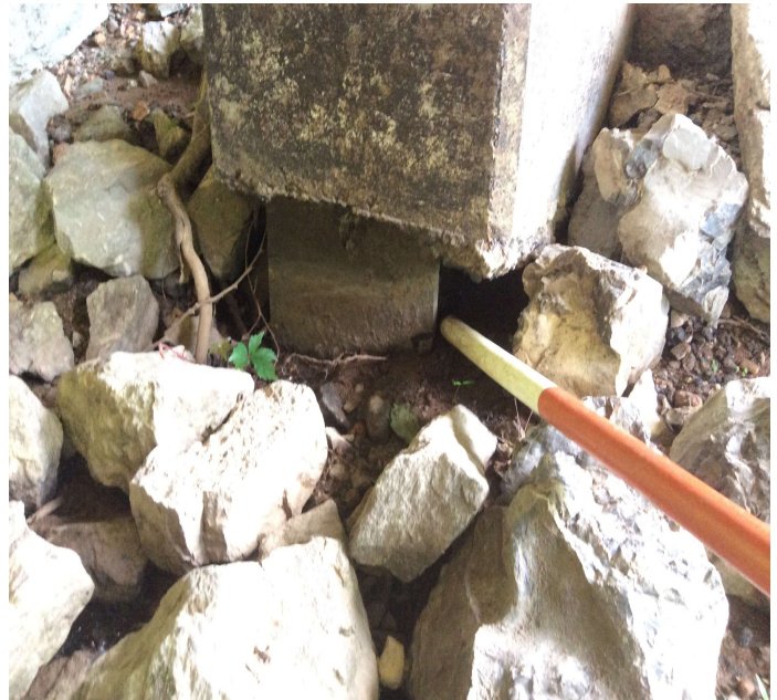
PHOTO 2 Description Bent 1 column 2 ahead side steel piling visible.
