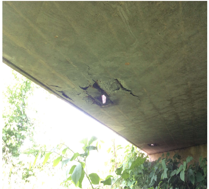
PHOTO 2 Description Span 3 left spalling around deck drains typical
