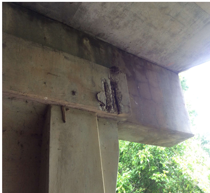
PHOTO 1 Description Spall with rebar exposed at ahead side of bent #2 upper right corner.
